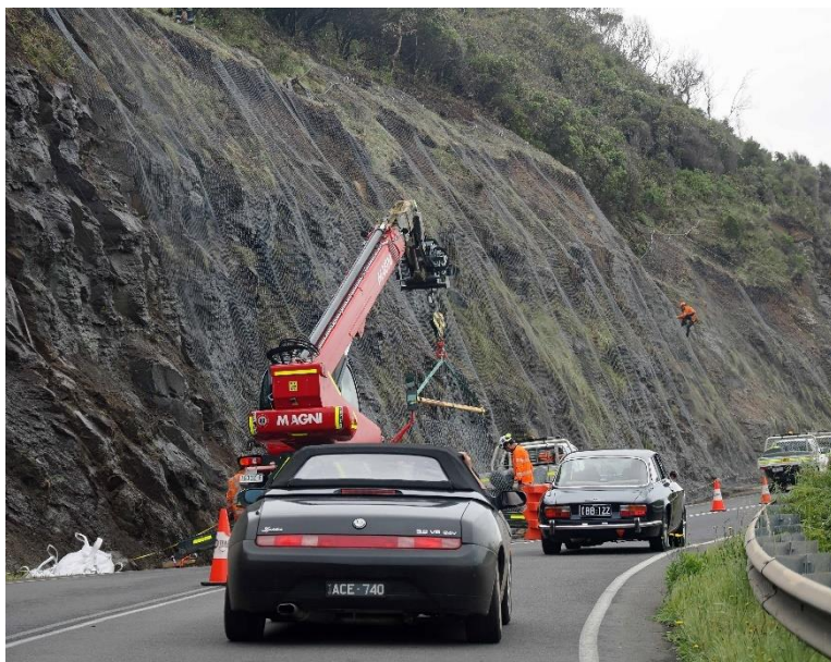
‘Netting’ being fixed to the rockface (Photo Andrea Sadow)
